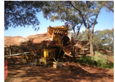
Gravity Recovery Plant
