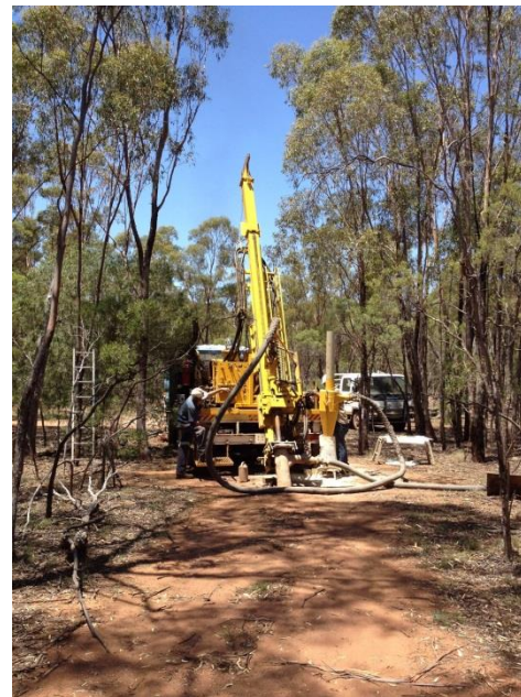
Drilling at the Gap Location
