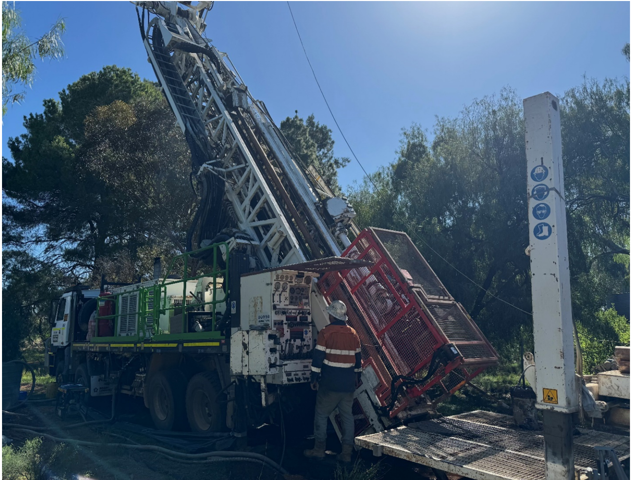
Figure 3: Murga Exploration Target – diamond drill rig set up on hole MS_DD2 (photo taken 11 December 2024)
