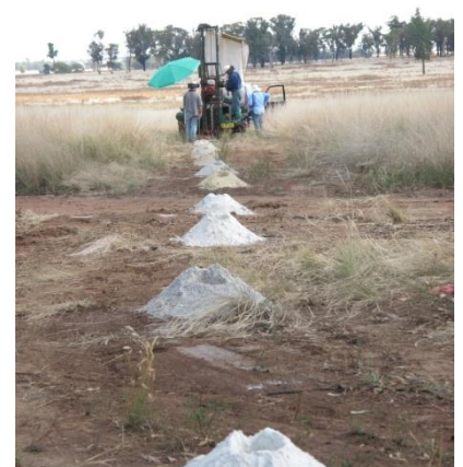
Auger Drilling into Bedrock 5m spacings
