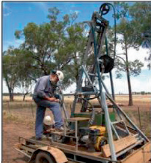
2 nd Auger Rig Operating
