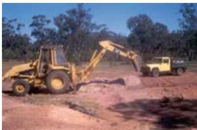
Trenching at Platina
